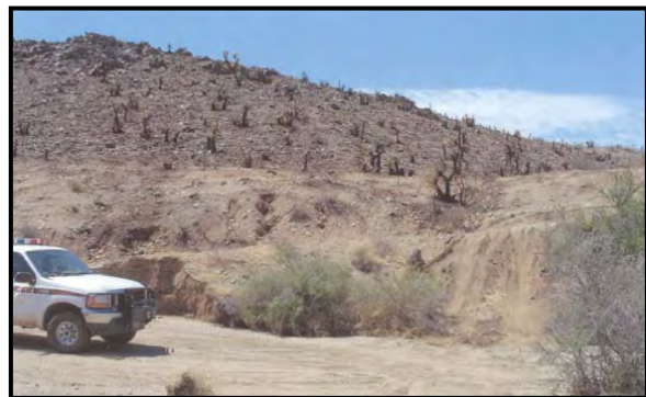
Unauthorized vehicle route in the Gold Butte ACEC
