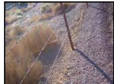
Standard 4-strand barbed wire fencing where tortoise-proof fencing material is attached
