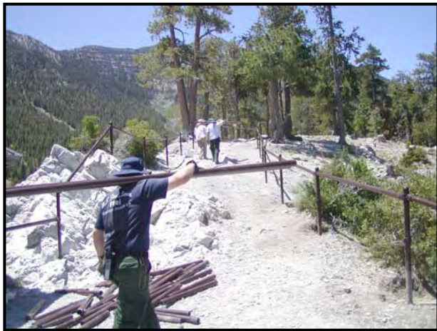
Fence installation in progress
